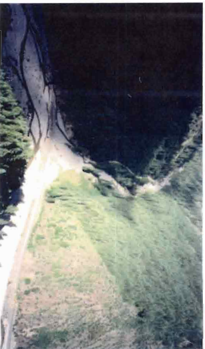
View of Highland Creek confluence. County Road acted as debris dam after undersized culvert clogged. Creek finally washed out road. Note large amount of stored sediment in creek channel upstream.
